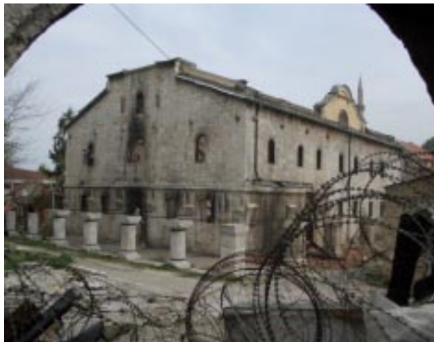
Not far from Judge Eisenhower’s residence, this Serbian Orthodox Church was surrounded by barbed wire fencing. The building had been burned in riots in 2004.
